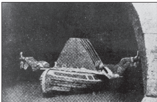
Legging in Islington Tunnel, c1916
